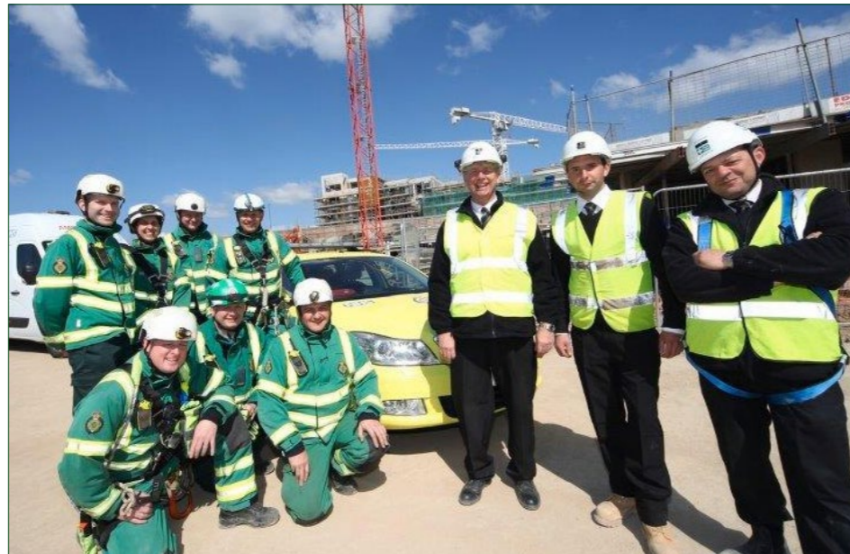
Pictured are members from the London Emergency Rescue team (far left) and CALA Homes at Millbrook Park construction team members: Tony Butcher (Project Manager), Alex Sgardea (Assistant Site Manager), Nick Taliotis (Site Manager)
